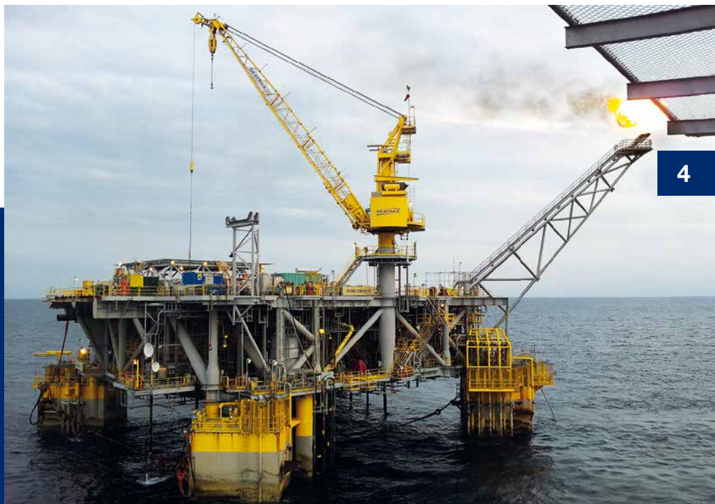
Tension Leg Platform with a 'Life support package' (blue Smit subsea container), which will be used to decompress divers in an emergency situation.
