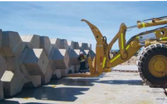
Offloading of 14.4t Xblobs from barge for installation into works
