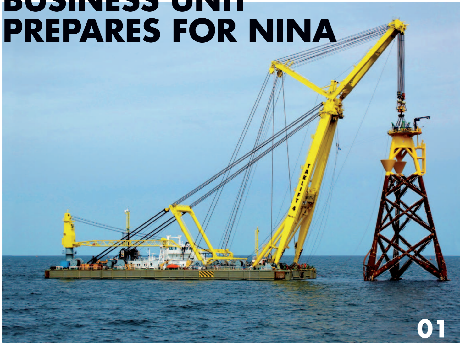
01 TAKLIFT 4 The sheerlegs Taklift 4 installing a jacket for an offshore wind turbine.
