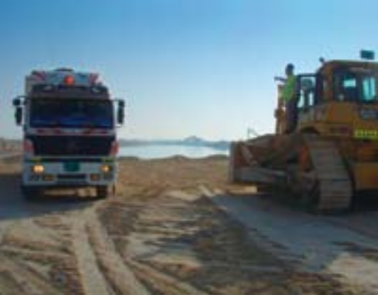
Bulldozer operator gives instruction in Khalifa
