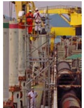
*Safety tops the agenda – scaffolding is erected for all jobs, including minor work, such as the inspection of a sensor above a bottom door cylinder.*
