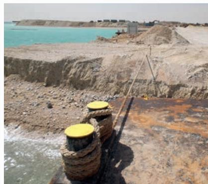
Snapback zone: if a line snaps, the sand dike will absorb the impact.
